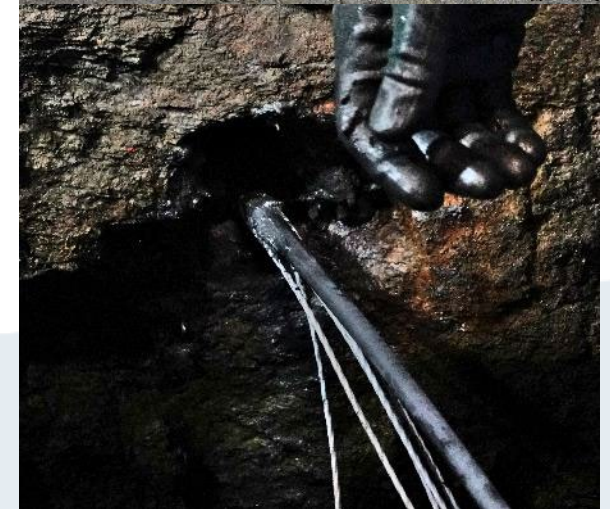
PT1000 sensors and sensor rod installation with thermocement
